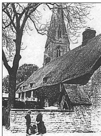
Former cottages at the Main Street end of Clatterpot Lane
