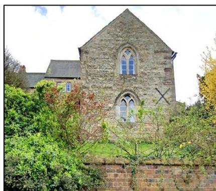
The north elevation of The Priory in 2026 (Google Earth).
