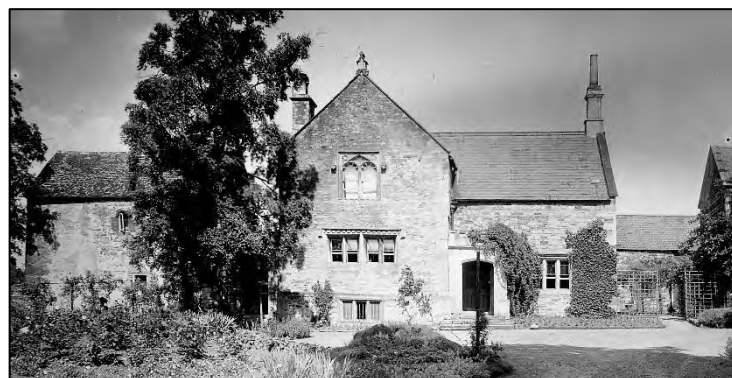
The Priory west elevation, about 1910 (Jack Hart Collection at Rutland County Museum ref 2002.6.0382).
