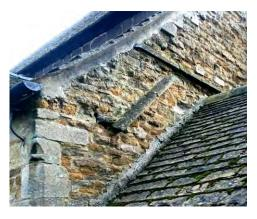
Fig. 37 (left). Indications of the slope of the roof of a now lost adjoining lean-to structure.
