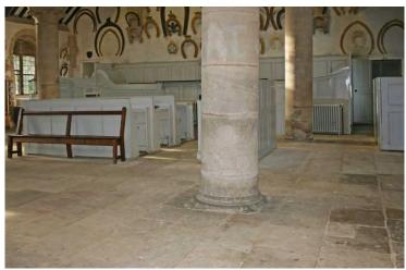
Fig. 24 (left). The floor at the west end of the Hall where it has been raised to the top of the column bases. The original floor level is that part of the present floor to the east of the two steps, which run across the building from north to south.
