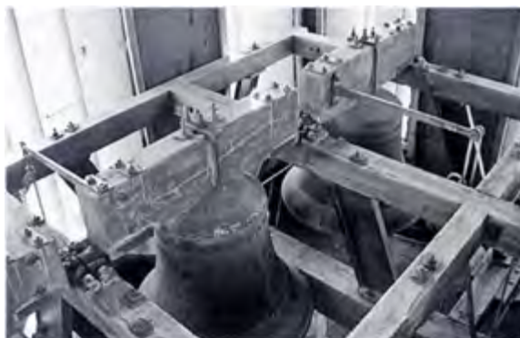
This photograph shows the third and fourth bells at Ketton. The construction of the composite frame installed in 1897 can also be seen. The canons were removed from all five bells when they were rehung at this time
