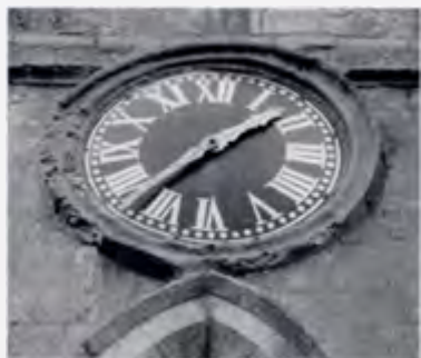
The present clock dial at Ryhall Church is on the north face of the tower. The dial surround was cast onto the face of the stonework
