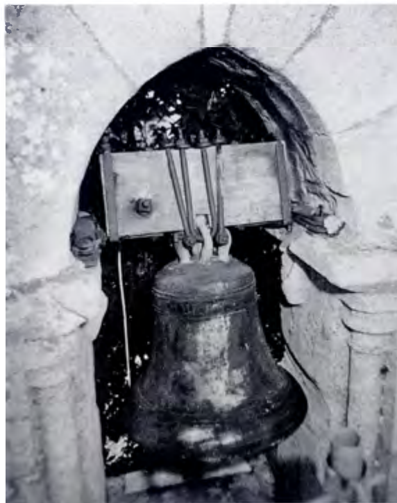
The treble at Pilton in its bellcote just before a new headstock was fitted in 1990 (Nicholas Meadwell)
