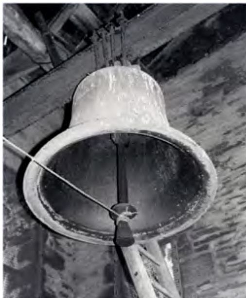
The Tixover bell is chimed from the base of the tower by a rope attached to the flight of the clapper. This is known as 'clocking'
