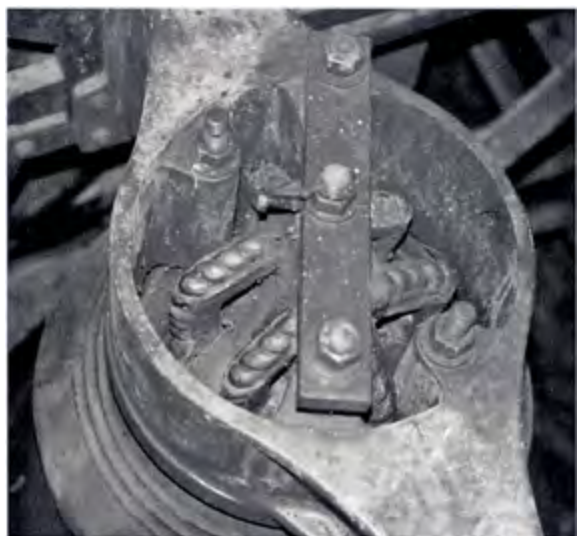
The canon-retaining headstock and decorated canons on the fourth bell by Thomas Eayre II at North Luffenham
