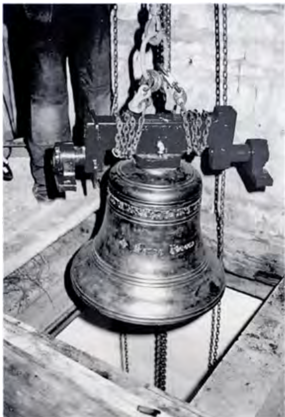
The new treble is hoisted into the belfry at Barrowden in 1990 (Nicholas Meadwell)
