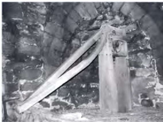
(right) Ryhall church clock. Showing how the clock weights were suspended prior to the clock being converted to automatic winding in 1979
