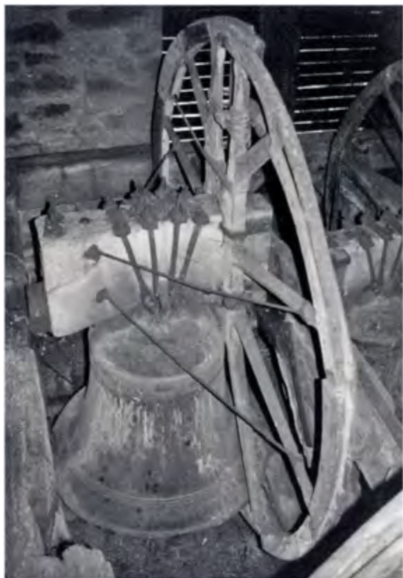
The tenor at Ryhall. Note the massive timber headstock and the unusual design of the bellwheel
