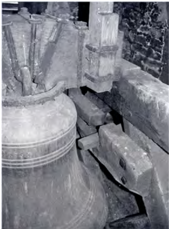
Unusually, the slider is pivoted outside the bellframe at Thistleton Church
