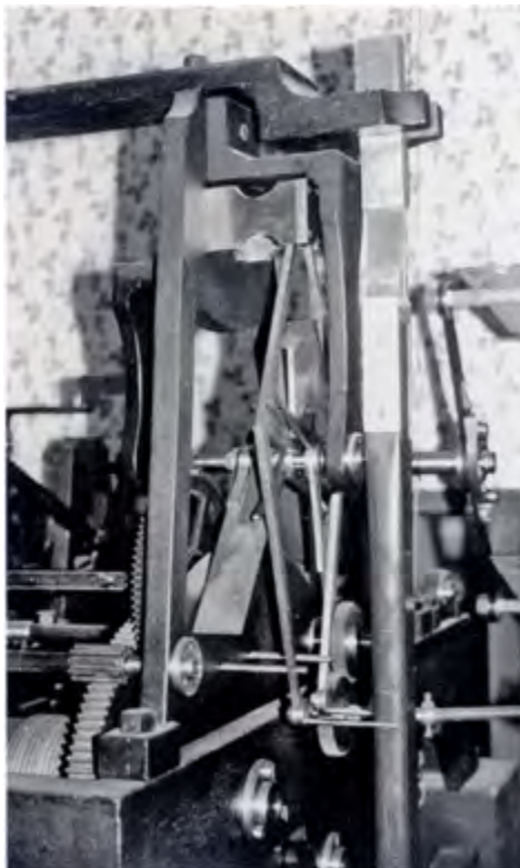
The double three-legged gravity escapement of the Stocken Hall Coach House clock
