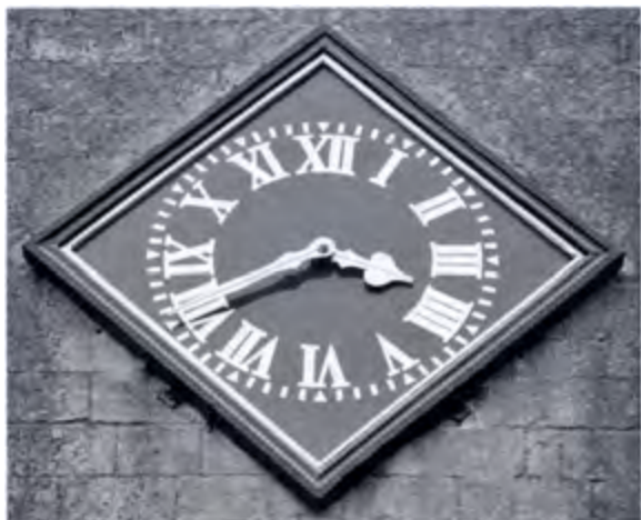
The clock dial on the north face of the tower at Ashwell Church in May 2000. It is based on the original early eighteenth century dial, although this would have been marked out for a single hour hand with quarter-hour divisions inside the chapter ring
