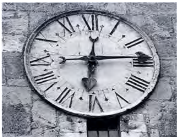
The dial installed by Henry Stone in 1775 at Edith Weston Church. The minute hand was added when the new clock was installed in 1928. The mark on the wall around the dial indicates that it originally had a stone bezel and this is confirmed by the circa 1793 drawing (RCM F10/1984/16)
