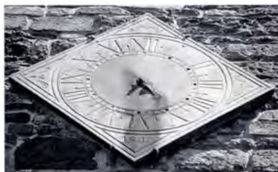
The slate clock dial on the west face of the tower at Stoke Dry. Note that it is marked out for a single hour hand, having four divisions between the hours
