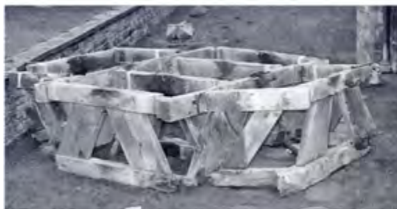
North Luffenham Church. When the 1701 frame was removed in 1984 it was temporarily reassembled in the churchyard (Nicholas Meadwell)
