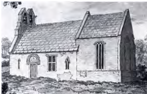
From a slightly later drawing of Essendine Church by Nathan Fielding showing that the structure had been removed from behind the bellcote and that the bells were rung from inside the church (RCM F10/1984/21)
