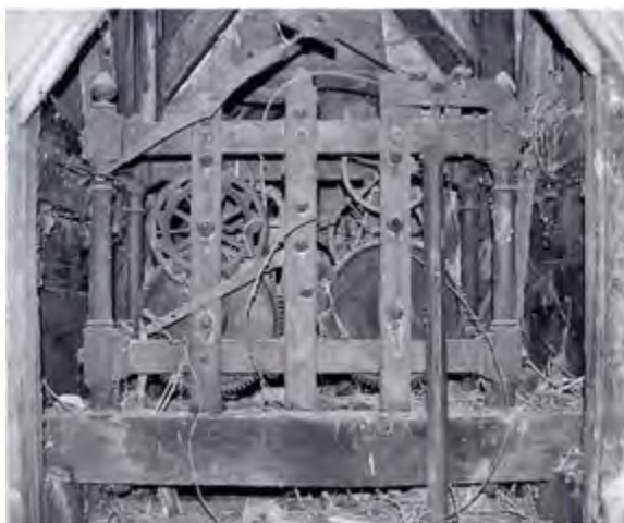
The posted frame turret clock by Alexander Simmons of Warwick in the former stables at Grange Cottage, Ketton
