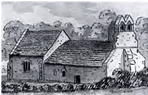
From a drawing of Essendine Church circa 1793 showing the structure on the eastern side of the bellcote. Such a structure would have enabled access to the bells from inside the church (RCM F10/1984/20)
