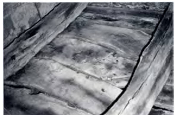
These floorboards were revealed when the old oak bellframe at North Luffenham was removed in 1989. They are the curved side members from the trusses of a circa 1500 frame (Nicholas Meadwell)
