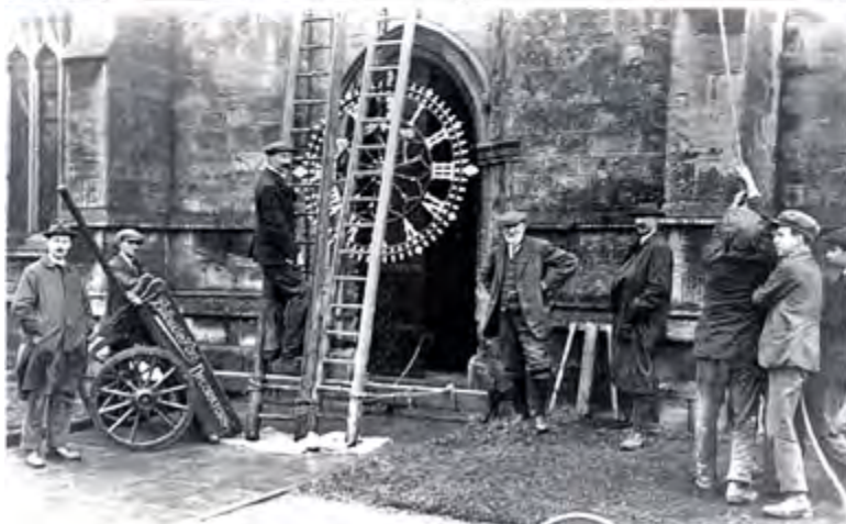
This photograph shows the newly regilded west-facing clock dial being hoisted back into position circa 1930 (DE 2694/241). As the handcart shows, the work was carried out by Billows & Son who had premises at 20 Northgate Street (Kelly 1925, 736). The dials were again regilded in 1993. This work was paid for by a grant from the Town Council as it is the only public clock in Oakham
