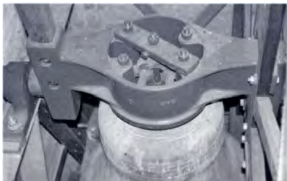
The canon-retaining headstock now fitted to the second bell at Brooke
