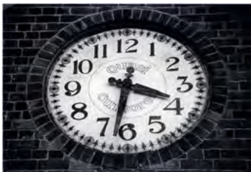
One of two slave dials of a Gent electric master clock system located in the physics laboratories of Oakham School, the other dial being located in the physics quadrangle
