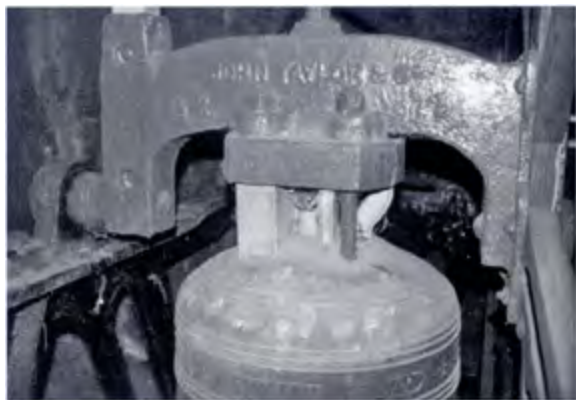
The canon-retaining headstock on the tenor at Glaston
