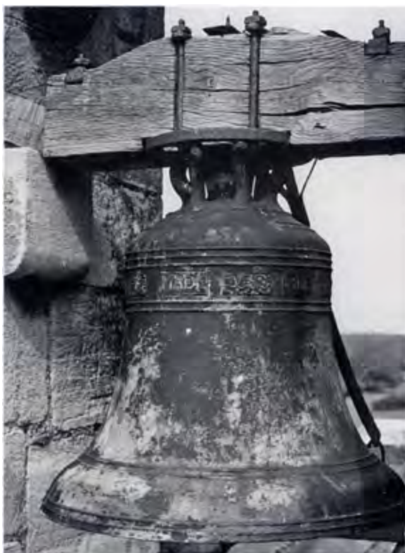
The Norris bell at Stretton Church showing the old headstock. In 1988, Nicholas Meadwell rehung both bells with new headstocks and bearings. The new headstocks are engraved NJM 1988 (Nicholas Meadwell)
