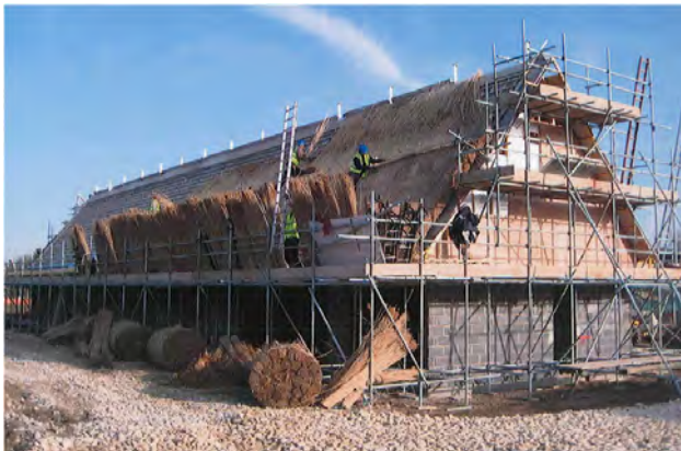
The new Rugby pavilion at Uppingham School Sports centre under construction
