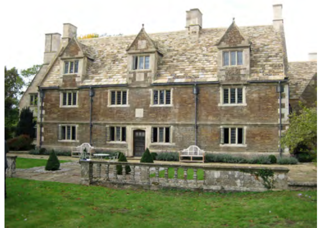
Langham Old Hall in 2011. It has been extensively restored following a devastating fire in October 2007. The fire swept through the roof and kitchen wing to the extent that the roof timbers were severely damaged, windows destroyed and stone walls left in an unsafe condition. Old Hall has a date stone of 1665, but its initial construction by Luke Sharpe was probably that of an important yeoman farmer's property rather than the building it subsequently became. Owen Hugh Smith acquired Old Hall in 1922 and employed the Arts and Crafts Architect H S Goodhart Rendel to create designs for extending and improving the building and its gardens, as well as providing a new entrance lodge and converting five cottages into a guest annexe. Most of the work was completed by 1926.
