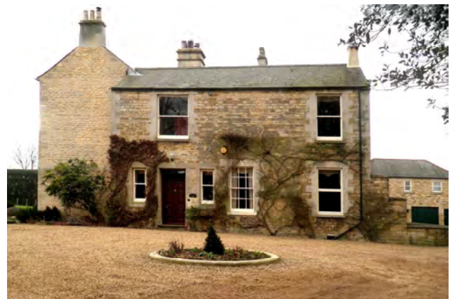
The east-facing elevation of Cottesmore Grange showing the new offices built for Richard Westbrook Baker in 1831.
