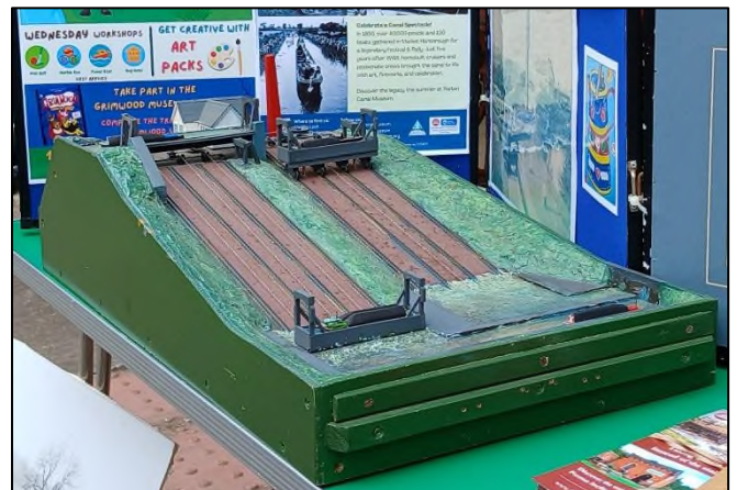
Foxton Canal Museum stand included a model and details of the inclined plane boat lift (RO).
