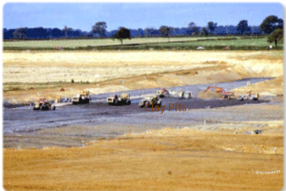
Building the dam wall
