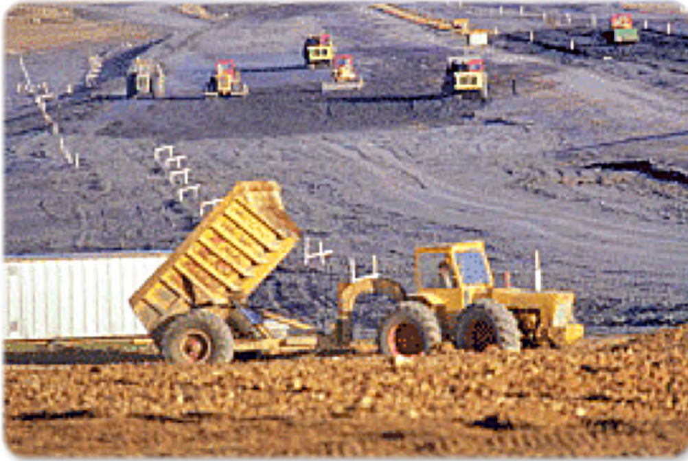
Building the dam wall
