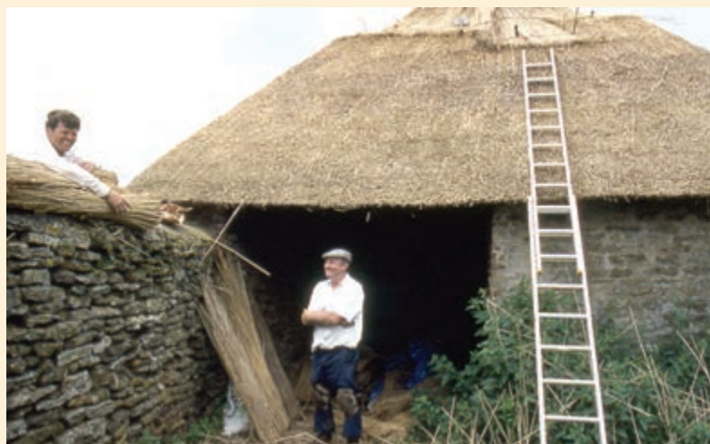
The Burley Hovel with its new thatch almost completed (TA)
