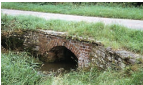
Above: Hobbs Bridge over the River Eg (Fred Adams)
