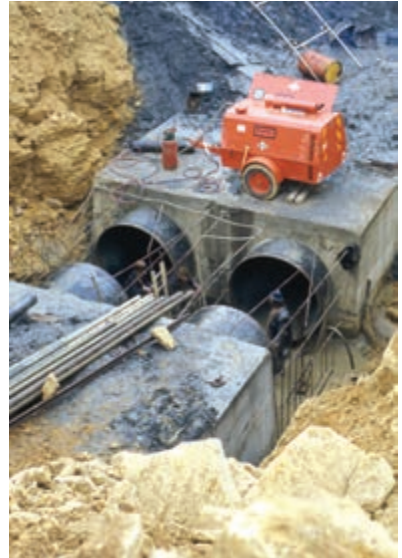
Above: Pipes were encased in concrete below the bed level of the River Welland (Brian and Elizabeth Nicholls Photography)
