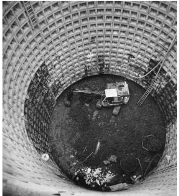
Above: Excavating the reservoir outlet shaft. It is 10.7m in diameter and over 30m deep (Brian and Elizabeth Nicholls Photography)
