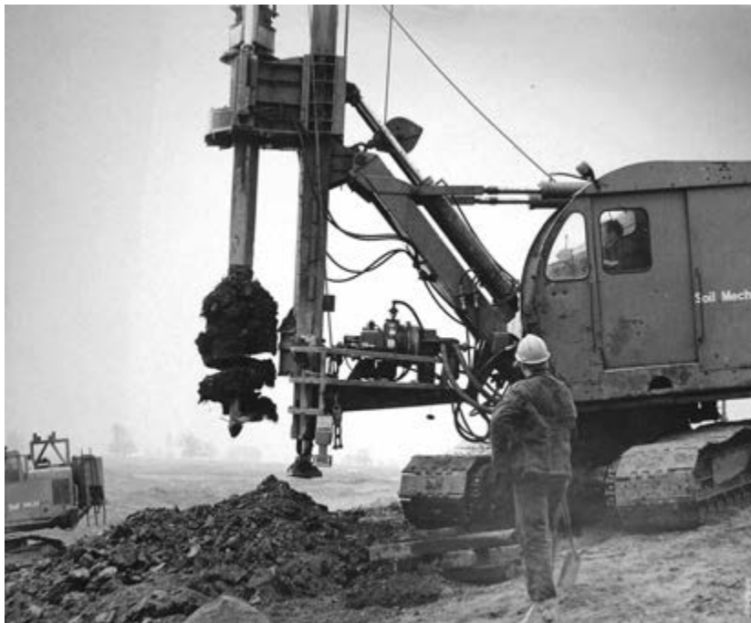
A crawler crane-mounted auger drilling a sand drain (Brian and Elizabeth Nicholls Photography)
