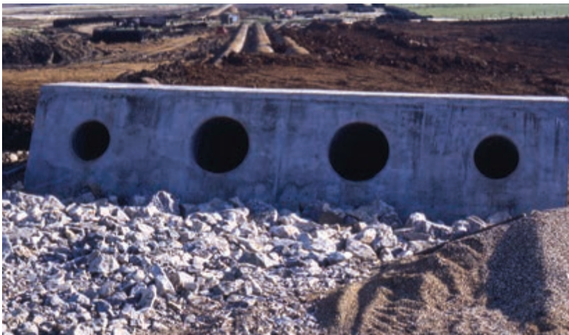
The four inlet jets pointing up the south arm of the reservoir (Brian and Elizabeth Nicholls Photography)
