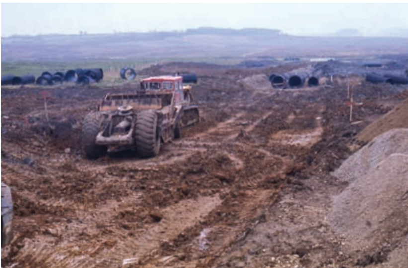
The four pipes to the inlet jets being installed across the valley floor near Normanton (Brian and Elizabeth Nicholls Photography)
