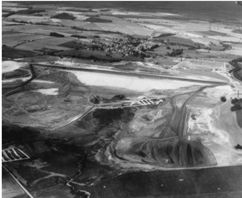
An aerial view of the borrow pits and the embankment, looking east towards Empingham (RCM)
