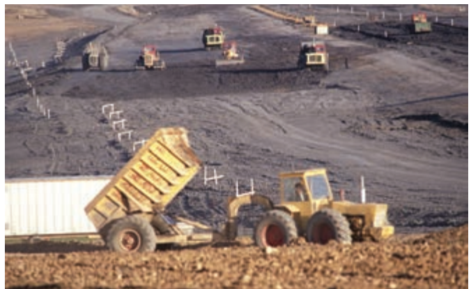
Spreading and compacting the clay at the south end of the embankment (Richard Adams)
