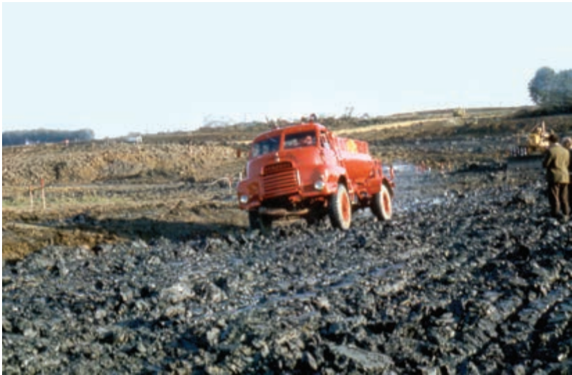
Watering the clay prior to harrowing and further compacting (Brian and Elizabeth Nicholls Photography)
