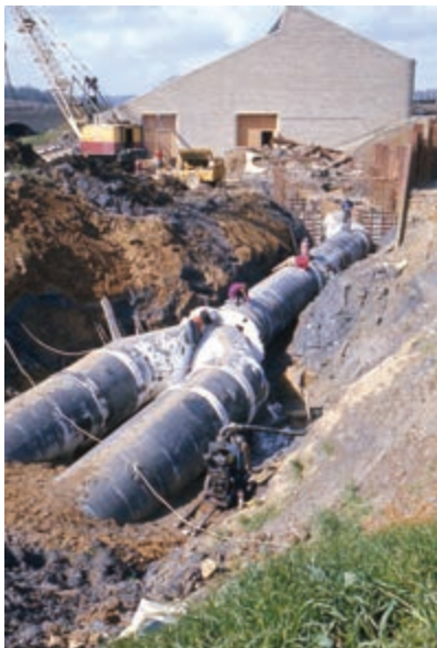
Steel pipes being installed near Wansford pumping station (Brian and Elizabeth Nicholls Photography)
