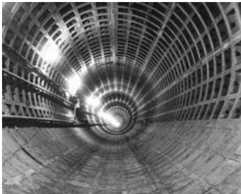
Above: The downstream diversion tunnel before the dividing platform was installed. It now carries the overflow water and other services (Brian and Elizabeth Nicholls Photography)
