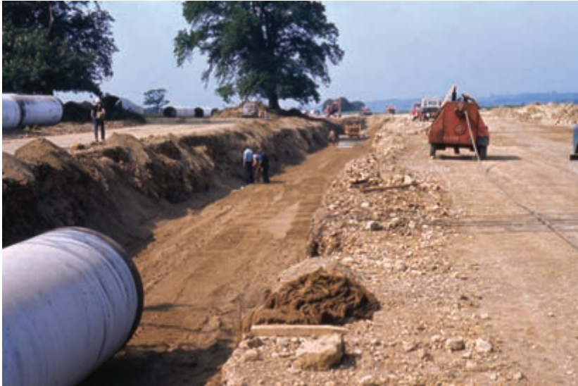
Installing the twin reservoir inlet pipes near Normanton (Brian and Elizabeth Nicholls Photography)
