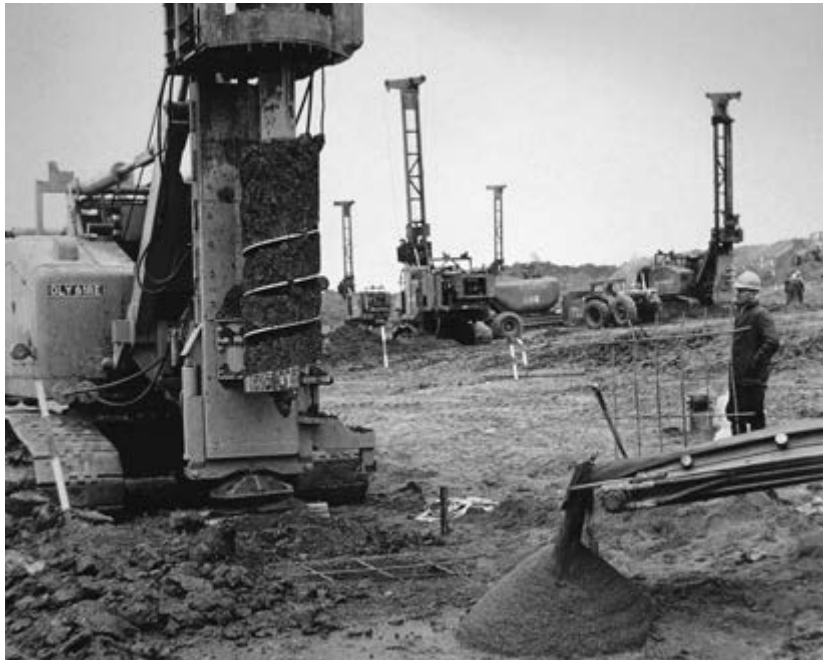
Installing sand drains in the foundation of the dam (Brian and Elizabeth Nicholls Photography)
