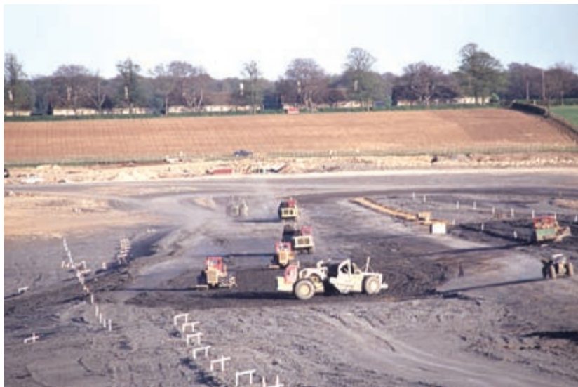
Left: Building the dam for Rutland Water in 1973 (Richard Adams)
