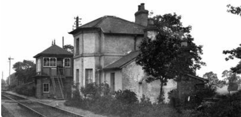
Egleton signal box and crossing keeper's cottage circa 1930. Both have since been demolished (May Wheatley)
