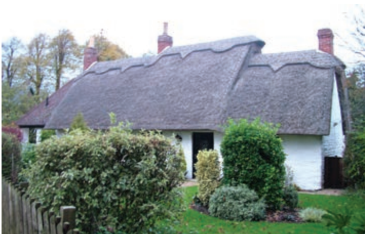
19 Church Road (4) in 1797 was home to Henry Towell, who was 'an old infirm cottager' who had 'built the Cottage himself' (RO)
